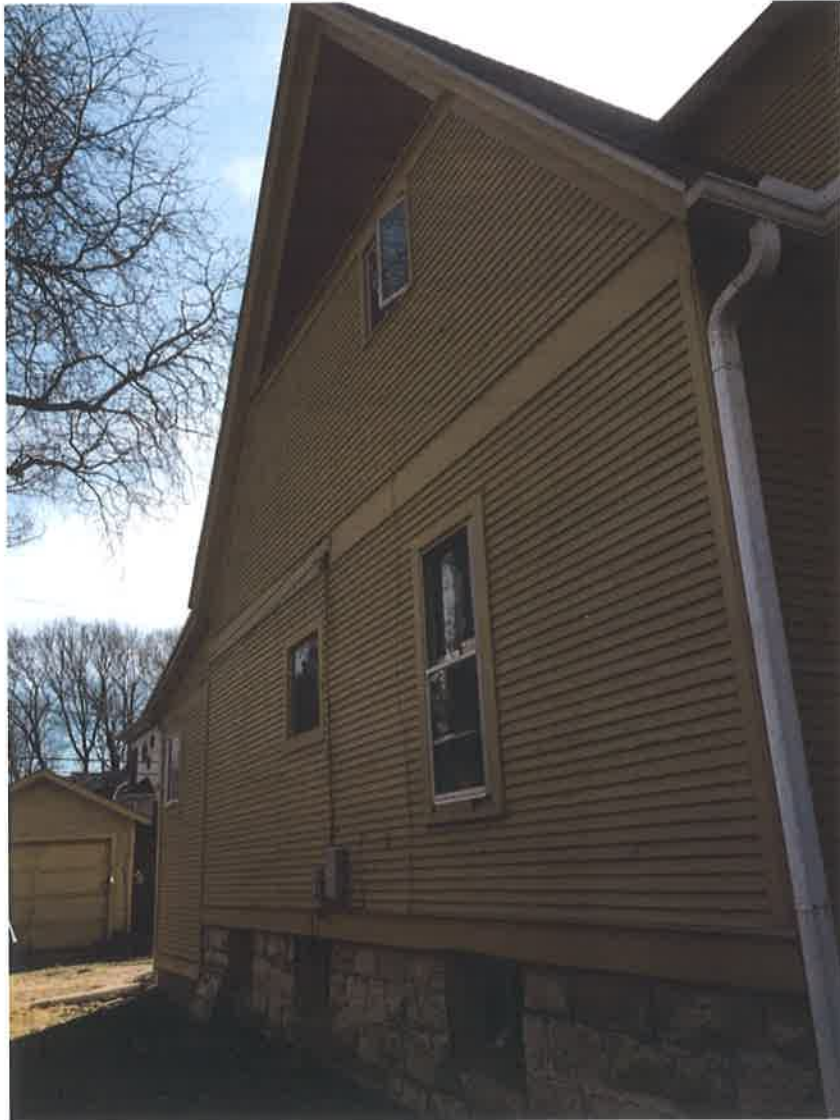
Photo #2: Side elevation facing north, April 2, 2019.
