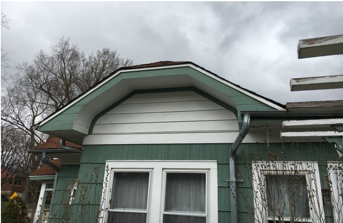
Photo #3: Jerkinhead (Clipped) Gable at South Elevation - April 4, 2017
