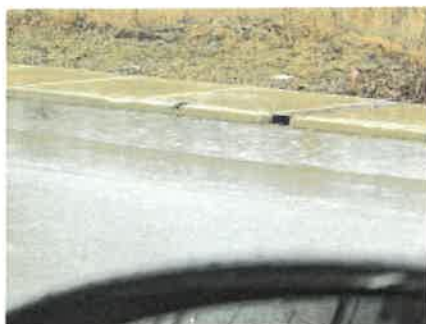
Drendel Road Flooded Street 2.jpg 2379K
