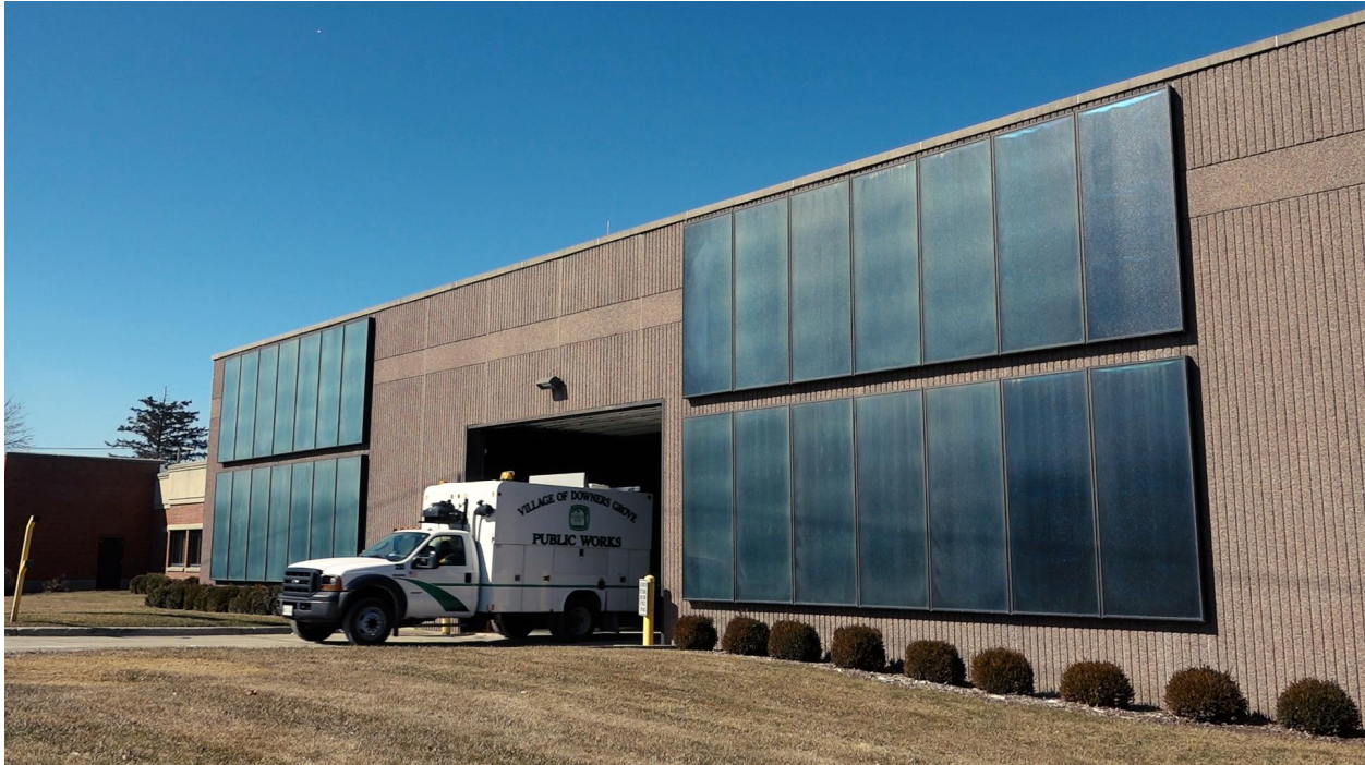
Solar panels on the Public Works building
