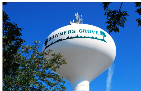
Elevated Water Storage Tanks
