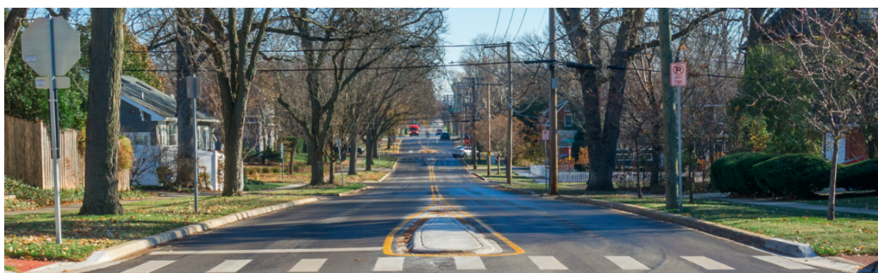
Recently Constructed Pedestrian Crosswalk on Prairie Avenue
