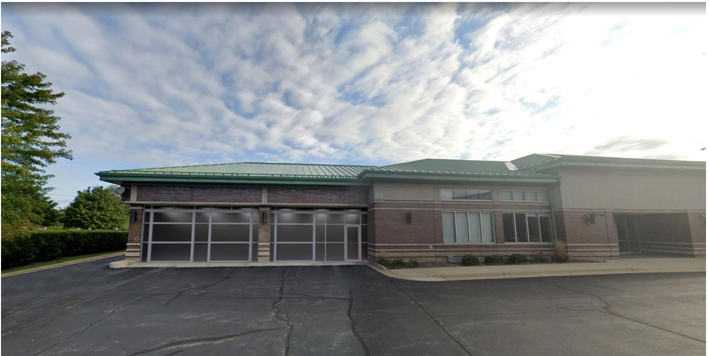
View from Wood Creek Drive looking north.
