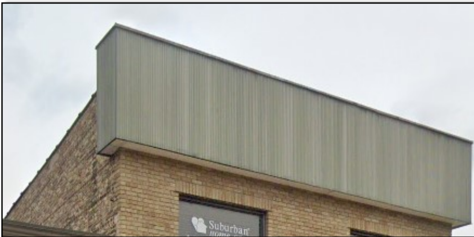
DISCOURAGED — Cornices should have detailing and should be in scale with the rest of the building. New cornices should not cover original features.
