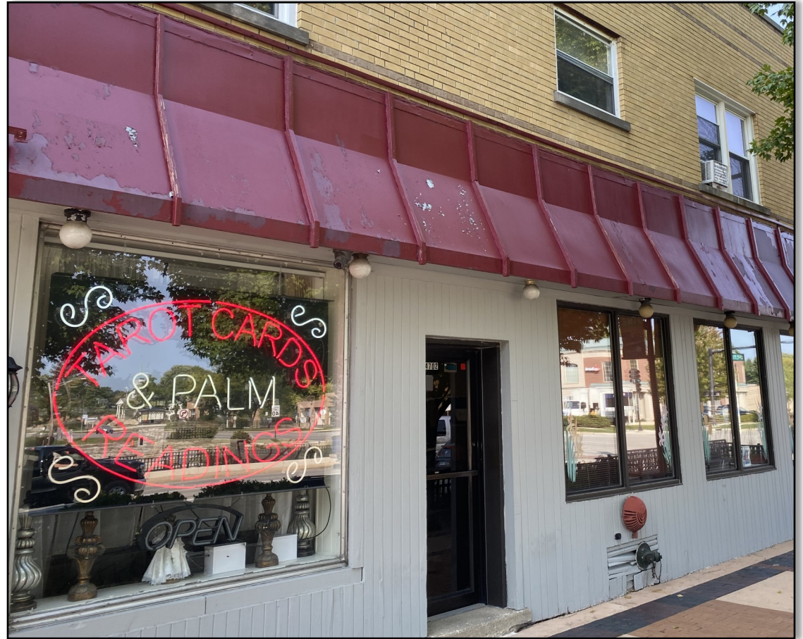
DISCOURAGED — Narrow and painted metal awnings lack durability and expose pedestrians to the weather.
