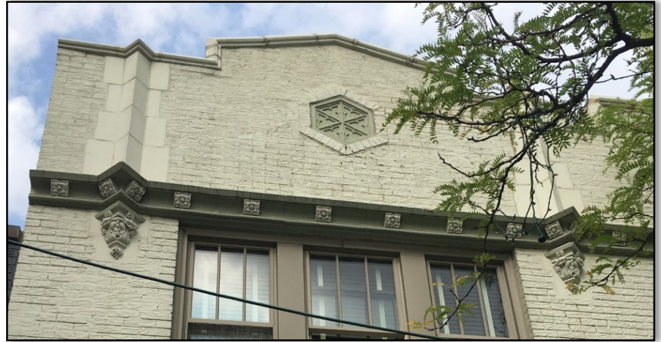
ENCOURAGED — Stone and cornice detailing.
