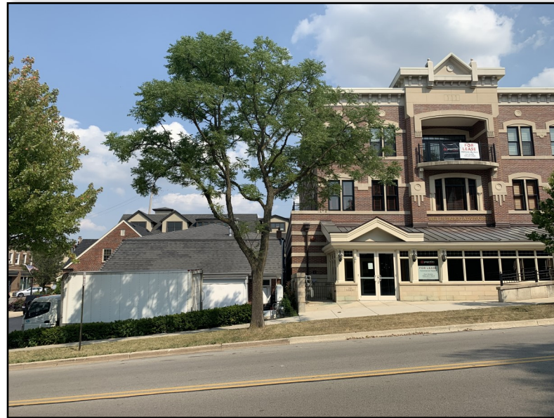
DISCOURAGED — Adjacent building should be complementary in height.
