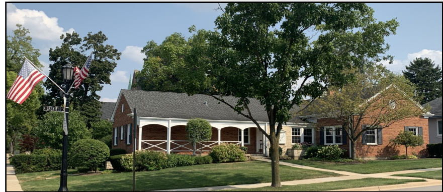
ENCOURAGED — Walkway from sidewalk to building entrance.
