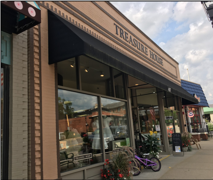
ENCOURAGED — Detailed knee walls and transom windows should make up a majority of the storefront.
