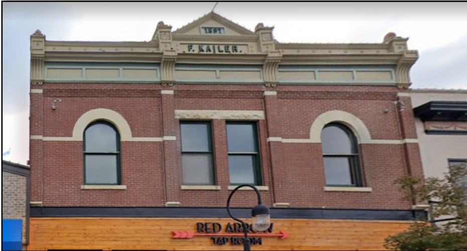
ENCOURAGED — Cornice detailing is in scale with the rest of the building.
