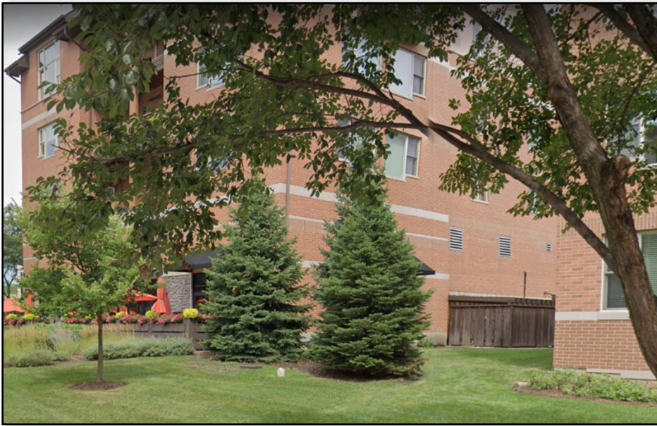
ENCOURAGED — Service areas should be screened where feasible with the use of extra landscaping.
