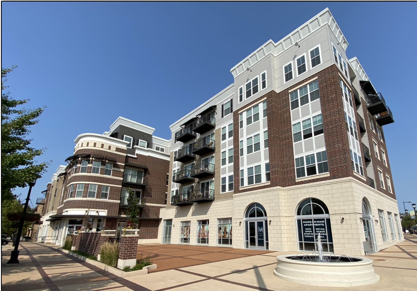
ENCOURAGED — Articulated middle with proportionate shapes and patterns. Inset and protruding balconies provide additional articulation.
