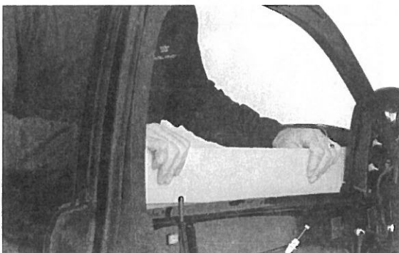
▲ Figure 27. Inserting the panel installation tool
