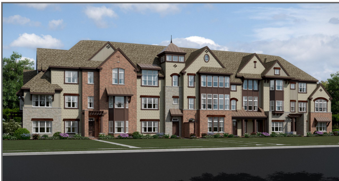
Similar project under construction in Libertyville
