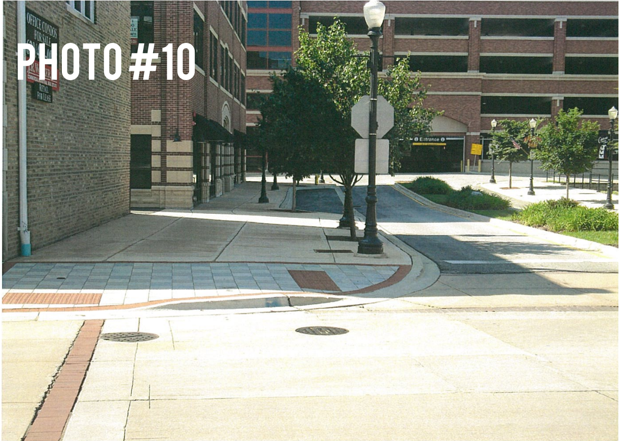
SE corner of Curtiss Street and Mochel Drive, looking south
