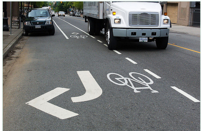
Demarcation on roadway for bicycle path and right turn lanes.
