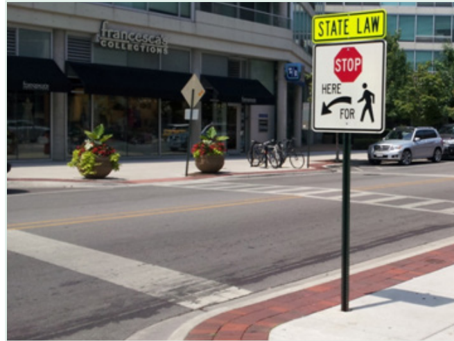
Example of Advanced Stop Line and Sign Utilization in Evanston, IL
