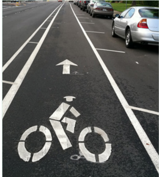
Example of a Buffered Bike Lane
