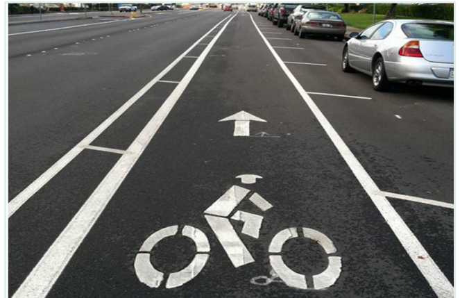
Many survey respondents were in favor of the utilization of buffered bike lanes to increase safety while biking in heavy traffic areas.
