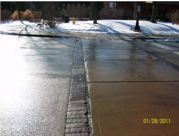
WARREN & HIGHLAND BEFORE
