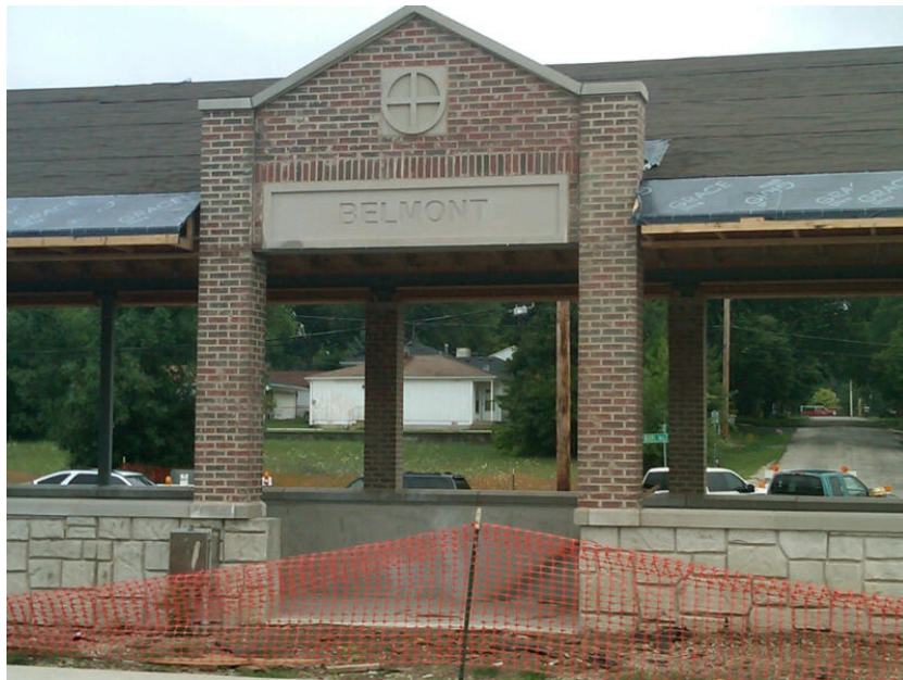
Pedestrian Underpass Structure Under Construction
