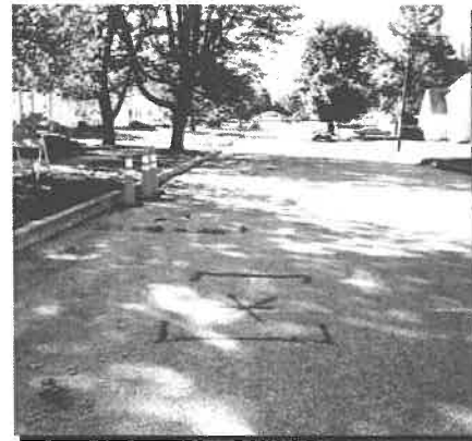
"X" marks the spot for excavation
