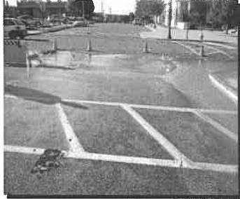
Leak surfacing at intersection
