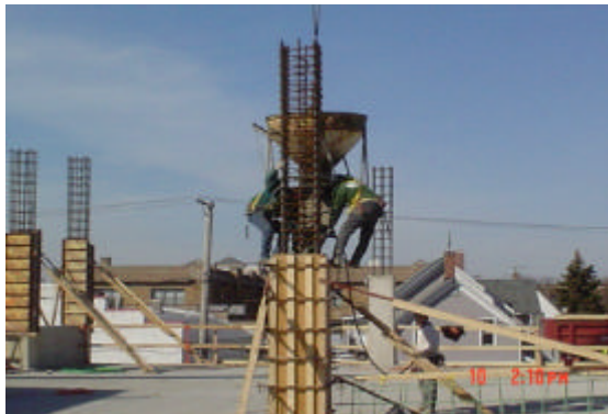
Placing concrete in columns, level 2 to level 3
