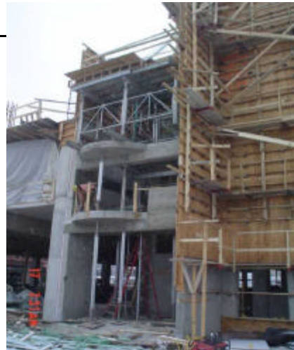
Stair/elevator tower #1 - Curtiss Street entrance
