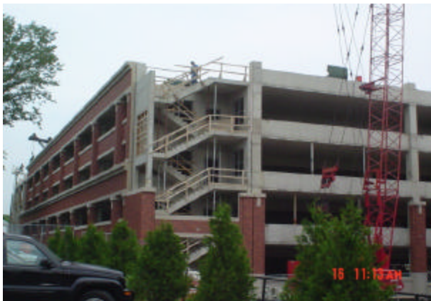
Southwest corner, looking northeast
