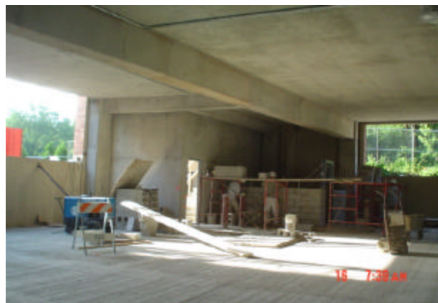
Building masonry wall for security equipment room
