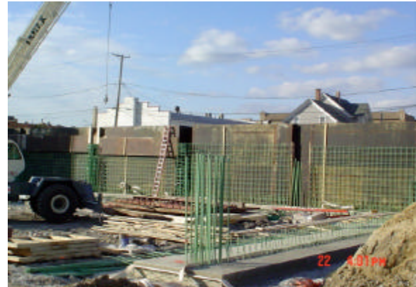
Formwork and reinforcing bars for north wall of detention basin.
