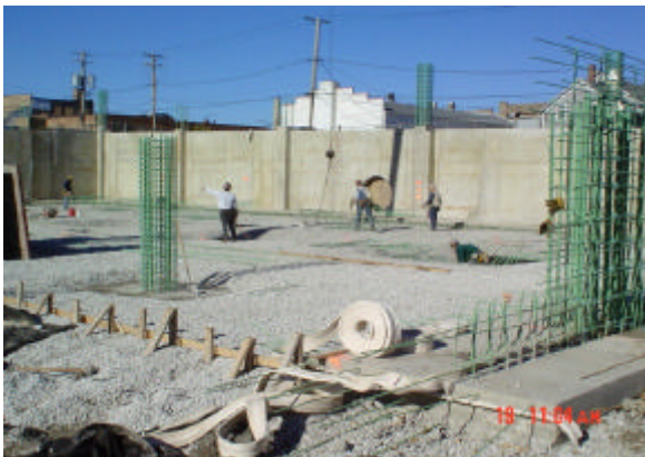
Placing rebar for detention basin slab (looking northwest)
