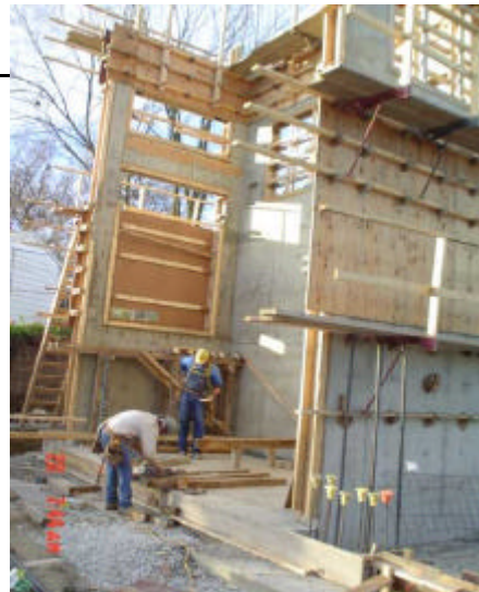
Forming stairs in southeast corner
