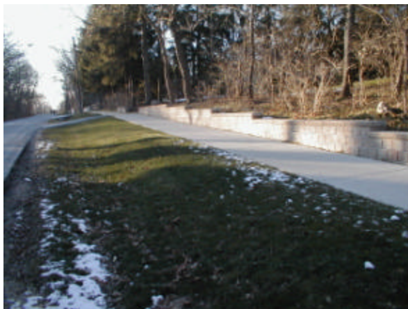
Chicago Avenue, just west of Downers Drive Intersection, looking West. Drainage ditch, sidewalk and Retaining wall.
