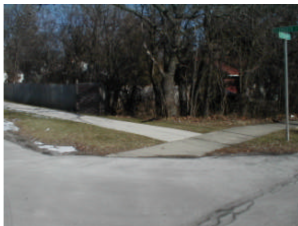
Plymouth & Jefferson Intersection, looking Northeast. New sidewalk connecting to existing sidewalk network.
