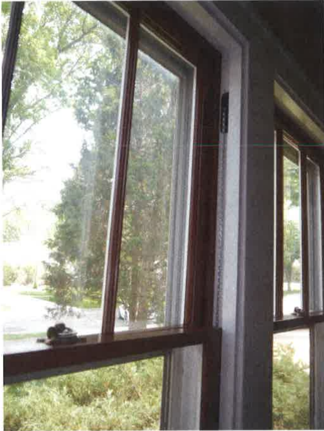
Photo #4: Restored window with new sash chain – June 28, 2015
