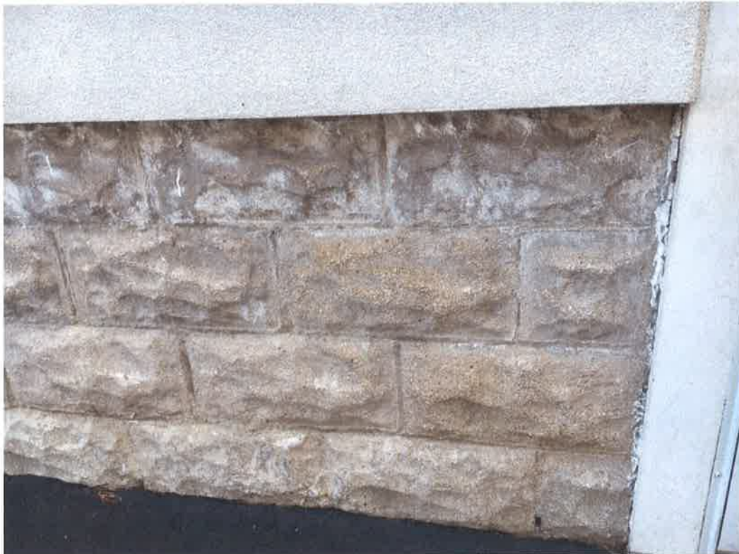
Photo #6: Rusticated concrete block foundation wall – January 10, 2016
