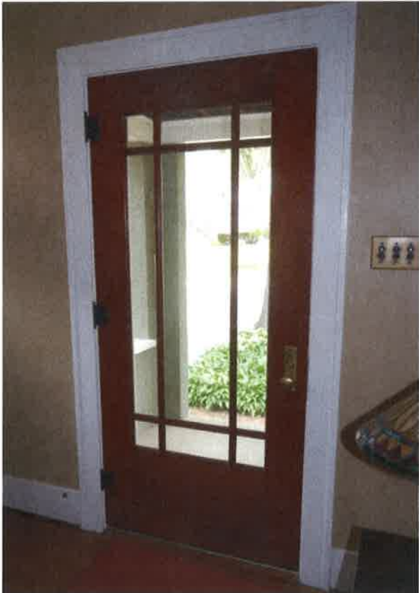
Photo #2: Restored Front door – June, 28, 2015
