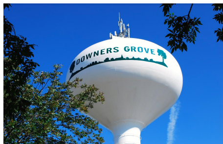
Elevated Water Storage Tanks
